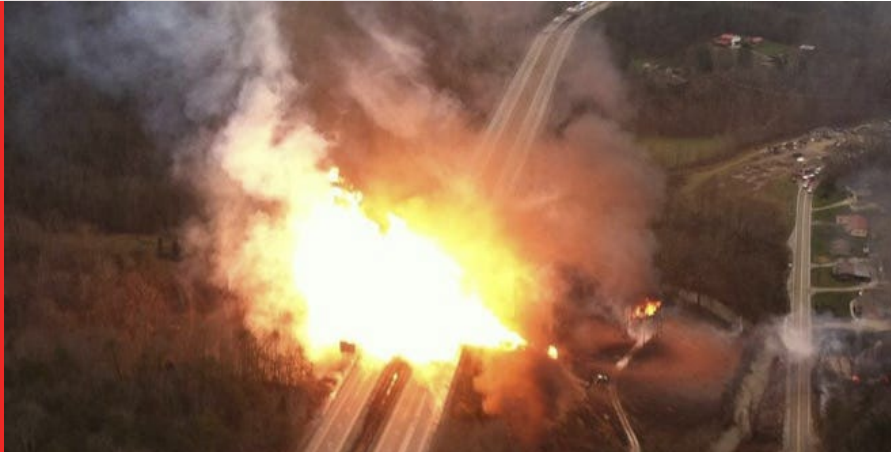
Gas pipeline explosion
